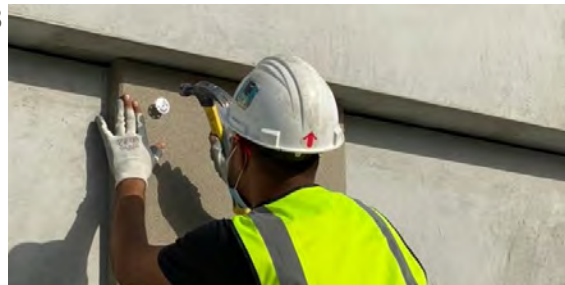
Gently hammer the pin in place
