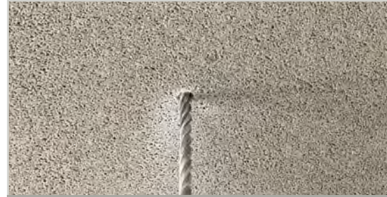
Drill into the centre of Reapor
