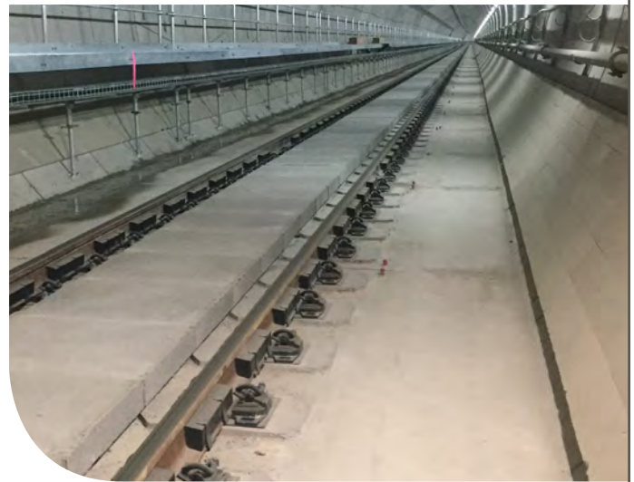
Viterolite® 900 in-between the rail track with Reapor on the wall
