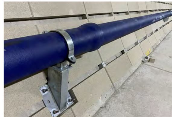
Tunnel application - Reapor installed on the wall
