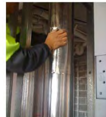
Tape all joints and edges for a tight seal
