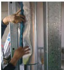
Wrap each segment with an overlap
