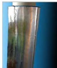
Tape along the longitudinal overlapped length
